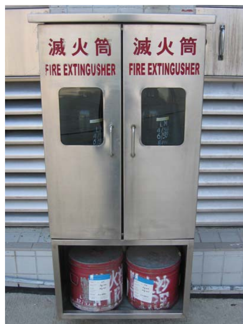
(Photo 8.2) Ensure all appropriate emergency equipment is readily available, i.e. fire-extinguishers and fire sand box.
